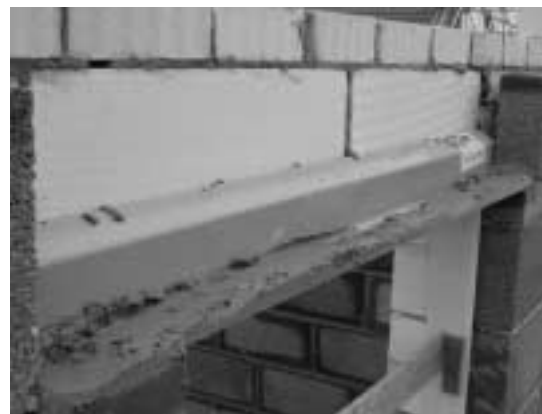
The Type C cavitray provides horizontal protection. Type L stopends prevent discharge into the cavity. Water is exhausted via caviweeps in the perp joints. The vertical cavicloser terminates tightly under the lintel.
