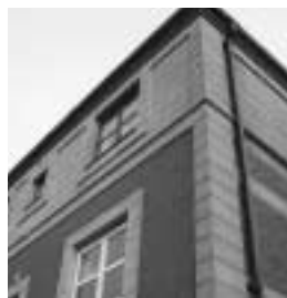
Cavity dropcloaks protect high-level dentil coursing and intermediate strings. The masonry bonding of the exterior skin is not interrupted. (1752)
