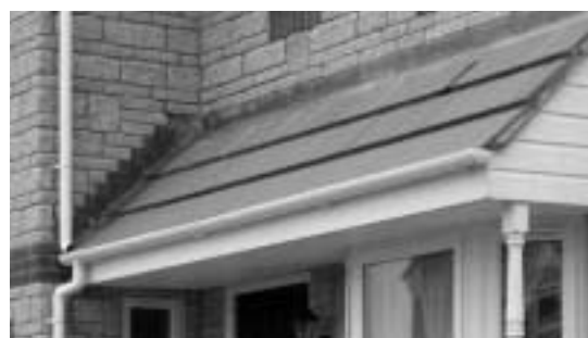
Type G provides the horizontal protection and Type X the stepped protection
