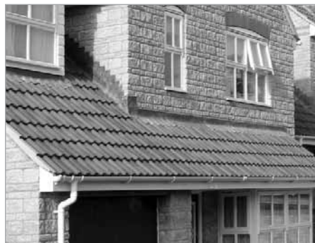
Type G Cavitytrays with attached lead flashings provide protection to the front horizontal intersection. Note the Type X cavitytrays used above the sloping abutment terminate with an external angle. This provides a protective link with the Type G cavitytrays.
