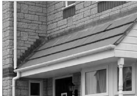
Type G Cavitytray provides the horizontal protection and Type X Cavitytray the stepped protection
