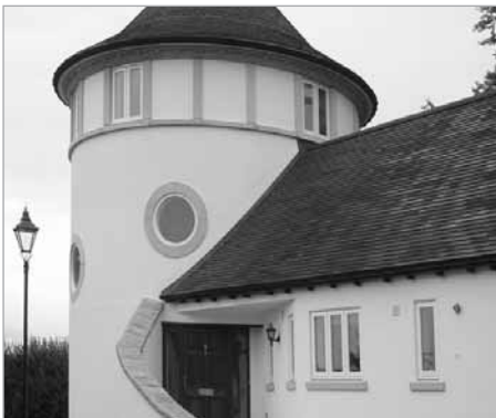
Typical example of gable abutment against convex masonry (see line drawing opposite).
