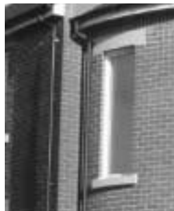
Curved lintel and curved masonry protected by cavitray of equal radius.
