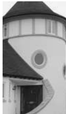
Typical example of gable abutment against convex masonry (see line drawing below).
