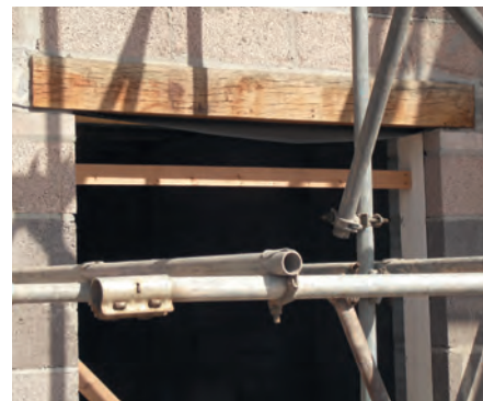
Opening ready to receive 2nd fix Quickcloser
